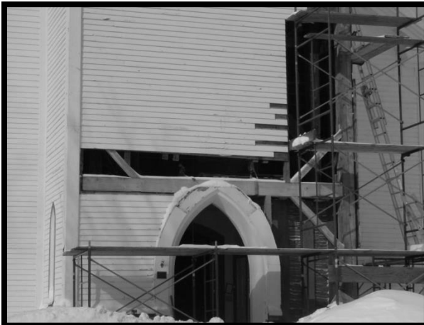
New plate with braces attached to new right front corner post. Tower Project 2011.
