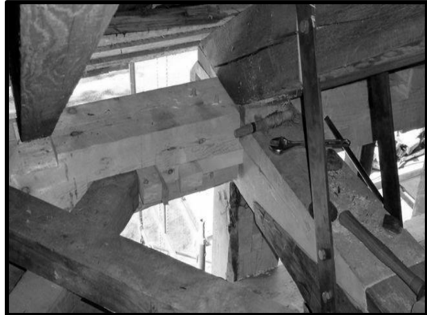
West Wall Timber Frame Repair 2015
