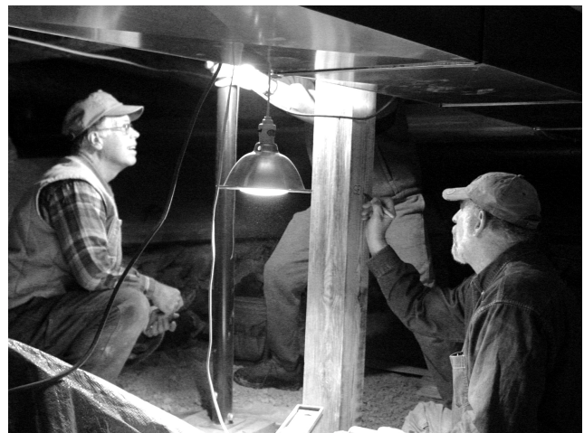
Pat Farmer and Bill McGroarty remove a jack, while Ken Secor puts the date on a new pressure treated replacement post.
